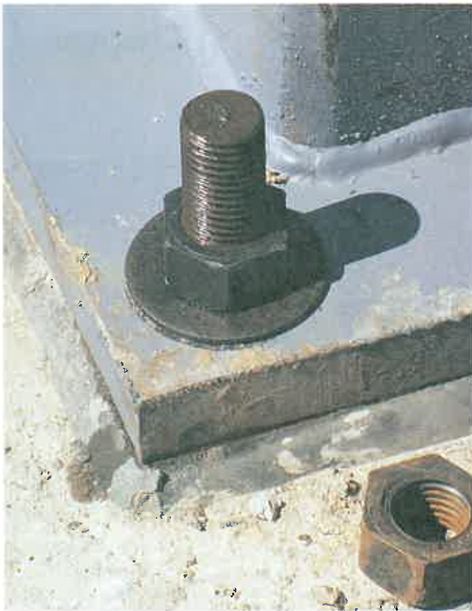
Figure 7-3. There is a wide range of threaded fasteners available, from tiny machine screws used in precision instruments to large bolts used in building construction. This 1" anchor bolt is being used to mount a steel column on a concrete foundation pier.
